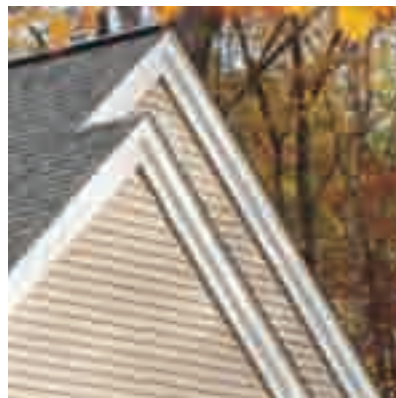
5" Trimworks lineals used as "rake" boards.
