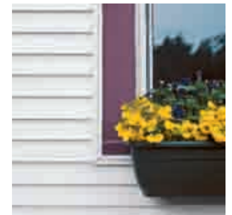
Trimworks custom crown molding used with wood window trim.
